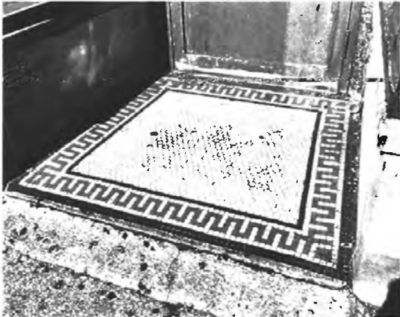
Figure 183. Acceptable example of historic storefront flooring
