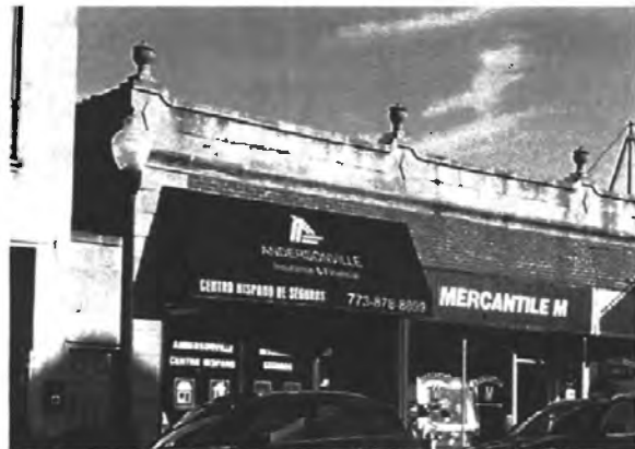
✗ Figure 186. Unacceptable example of replacement awning as it is not located within the existing masonry opening
