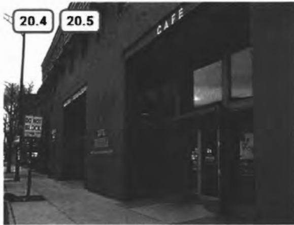
✓ Figure 77. Acceptable example of deeply recessed storefront and entry
