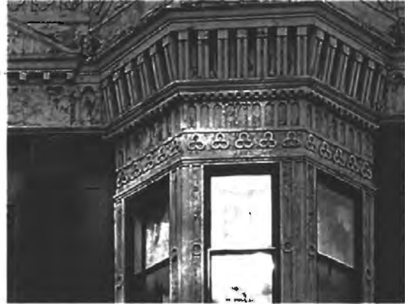
Figure 34. Example of character-defining, historic, architectural metal
