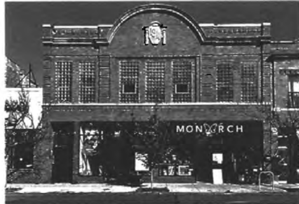
Figure 19. 2875 N Milwaukee Avenue
