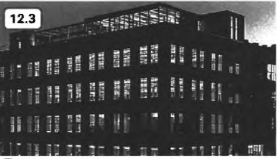
✓ Figure 58. Acceptable example of a design for an addition to an existing building
