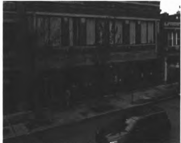
Figure 17. Sidewalks along Milwaukee Avenue (Scott Shigley)
