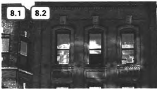
✓ Figure 48. Acceptable example of new windows in preserved masonry openings
