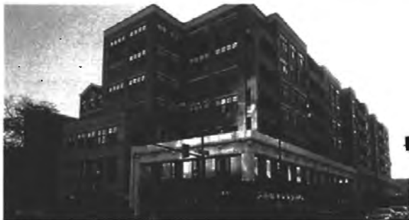
✓ Figure 40. Acceptable example of a facadectomy
