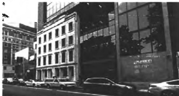
✗ Figure 43. Not acceptable as the upper floors of the new construction are not adequately setback from the historic facade
