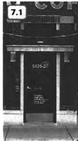
✓ Figure 45. Acceptable example of a replacement door in a historic opening
