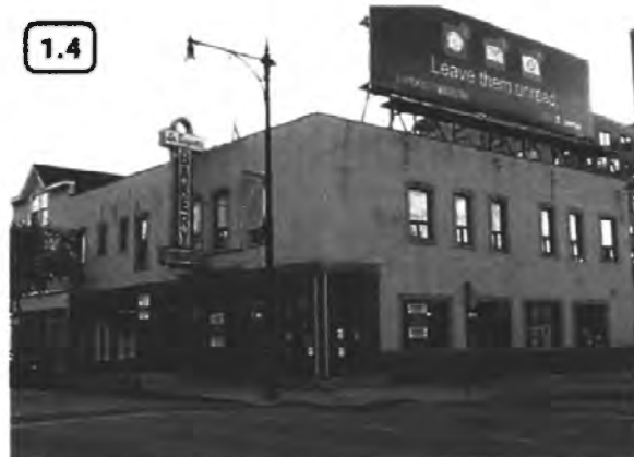
✗ Figure 33. Unacceptable cladding over existing masonry
