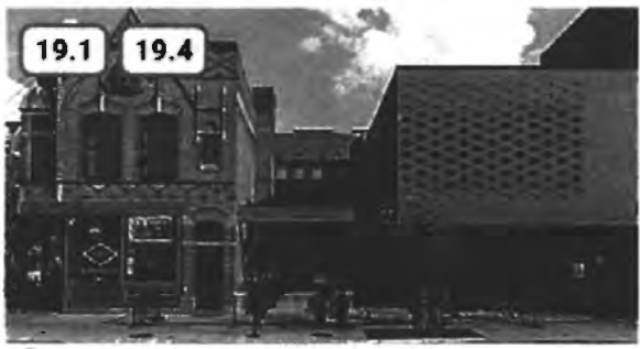
✓ Figure 70. Acceptable example of new material, texture, and articulation used at a primary facade of new construction that compliments the historic built environment
