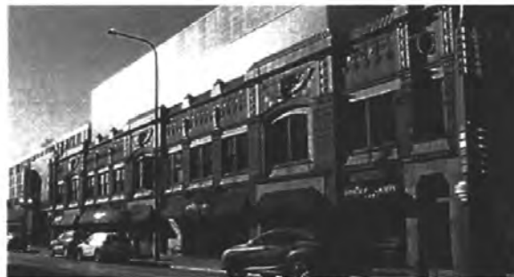
✓ Figure 42. Acceptable example of a facadectomy
