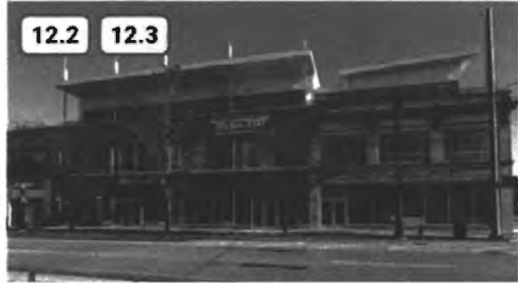
✗ Figure 59. Unacceptable example of an addition as the addition has a projecting roofline that does not minimize its visibility (Apartments.com)
