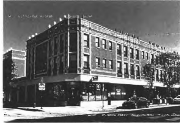
Figure 118. 2741 N Milwaukee Avenue
