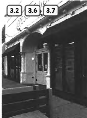
✓ Figure 38. Acceptable example of a new storefront that retained character-defining features of the original storefront
