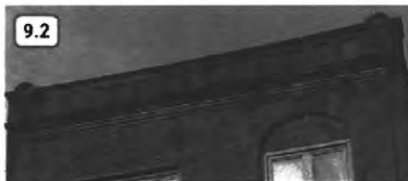
Figure 52. Examples of existing cornices in the district
