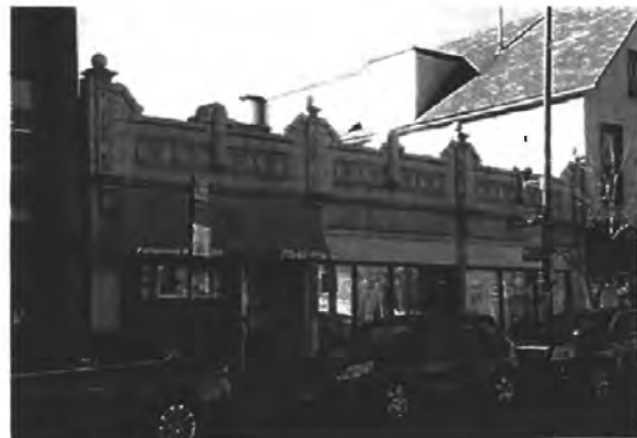
Figure 21. 2832 N Milwaukee Avenue
