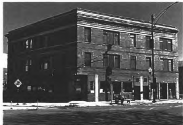
Figure 119. 2171 N Milwaukee Avenue
