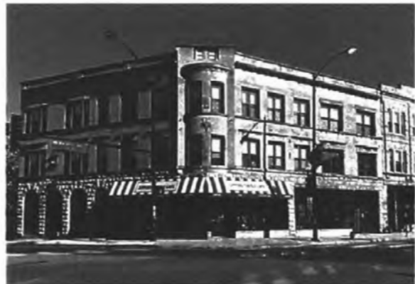
Figure 120. 2959 N Milwaukee Avenue
