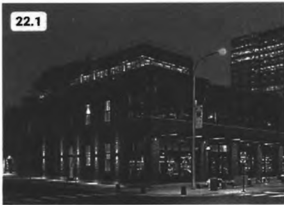
✓ Figure 82. Acceptable example of exterior building lighting
